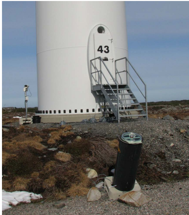
Figure 59. Camera system installed in connection to wind turbine no 43. Photo: Kjetil Bevanger.
