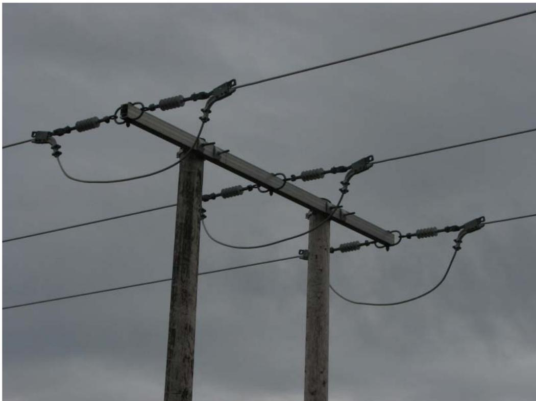
**Figure 19c.** *Pylon no 140. Metal cross-arm.* Photo: J.O. Gjershaug.
