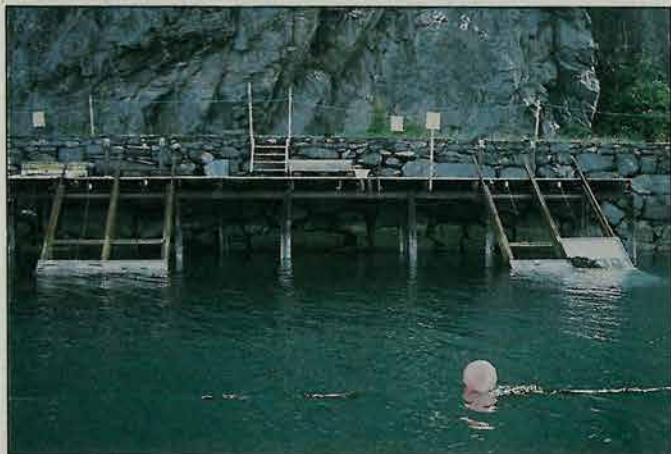
Figur 4 Sjøanlegget ved Institutt for marinbiologi, Universitetet i Bergen. - The experimental shore constructed at the Department of Marine Biology, University of Bergen.
