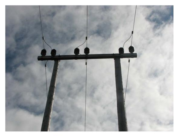
Figure 19h. Pole no 177. Double pin-isolator. Photo: J.O. Gjershaug.
