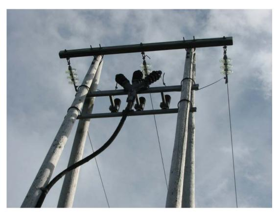
Figure 19i. Pole no 184. Cable debranching. Photo: J.O. Gjershaug.
