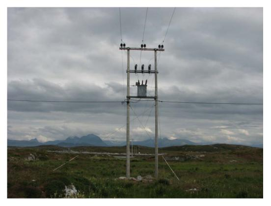
Figure 19e. Pole no 149. Pole-mounted transformer. Photo: J.O. Gjershaug.
