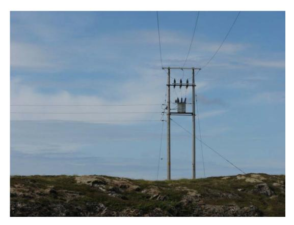
Figure 19j. Pole no 186. Pole-mounted transformer. Photo: J.O. Gjershaug.
