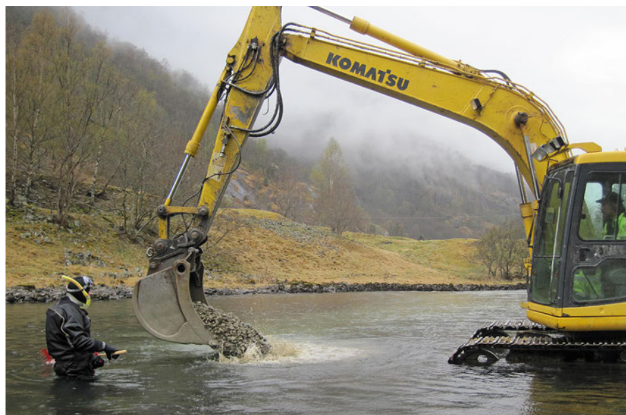
Figure 16. Installing spawning gravel using an excavator (from the Aurlandselva river in Norway). Trained personnel in snorkelling gear guide the operator as to volume and location, and then spread the gravel using scrapers and rakes. Photo: Bjørn Barlaup
